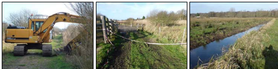
Digger on the permissive path; closed path; after ditching work
