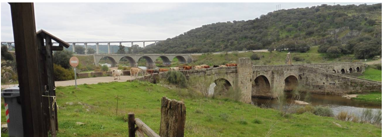
Three bridges over the Almonte River.
